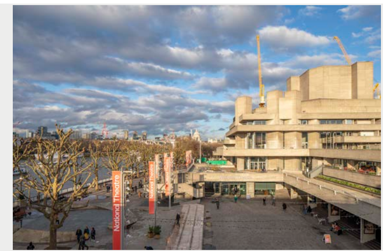
c32 | Waterloo Bridge downstream - overlooking terraces of RNT
