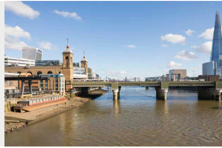
c12 | Southwark Bridge: downstream - close to the City of London bank
